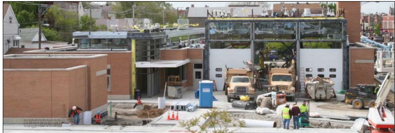
Construction site of the new Engine Company 109.
