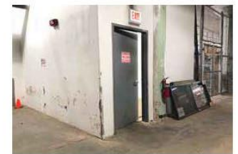
E - Condition at Exit 6
