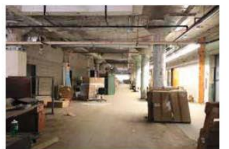
B - Circulation space between column lines 11-12
