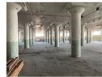
A - South side of floor
