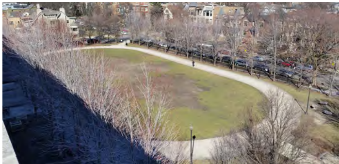
The site of Lake View's turf field before the renovation.
