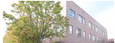
Edwards Elementary School Annex LEED Silver
